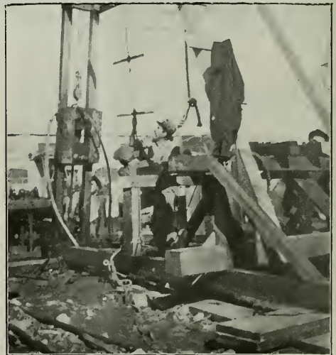
"A" Frames for Handling Steel. Note Movable Wood Block Carrying Jack-Hammer.
